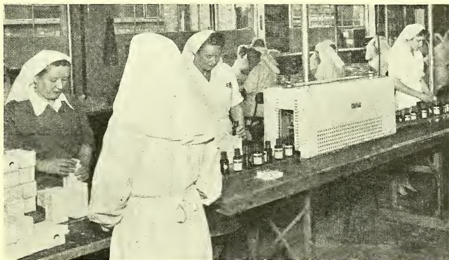
Drying bottle caps by infra-red heater.
